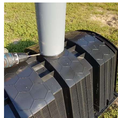
11. Install a stack
