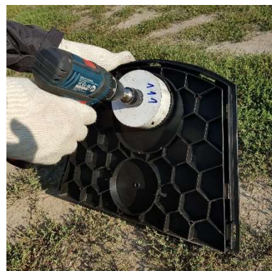
3. Drill a hole
