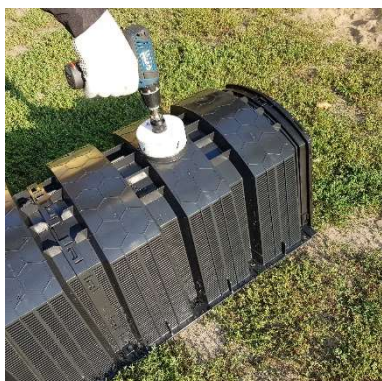
10. Drill a hole on the ridge
