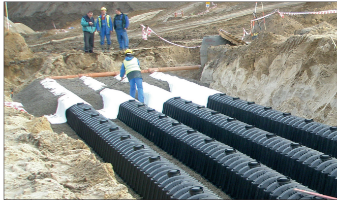
Figure 7 Installation of infiltration tunnels
